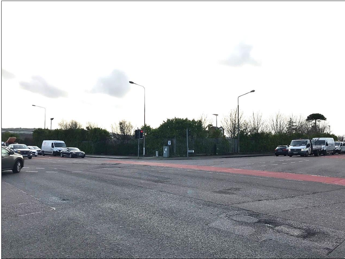
Figure 5. View of the site from the north-east at the junction between Kinsale Road (left middleground) and Tramore Road (right middleground).
